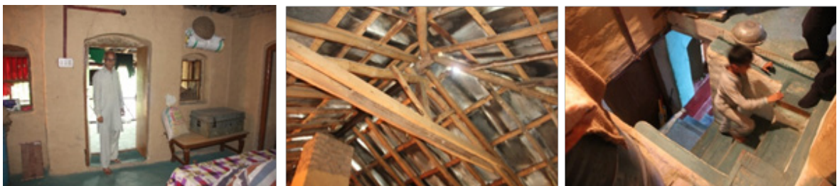
Figure 13 Features of vernacular house at Rajiana: a) Low ceiling Heights b) Truss with tie beams and c) Internal staircase for heat retention bracing made of local wood
