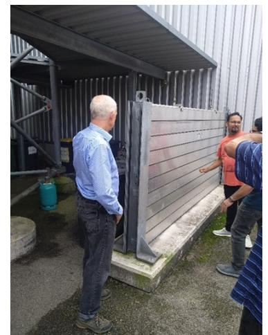
**Columns and plates used to construct walls**
